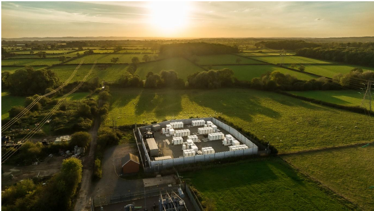
Photo Credit: Pulse Clean Energy
